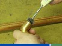
Cleaning the inside of a copper fitting prior to soldering.
