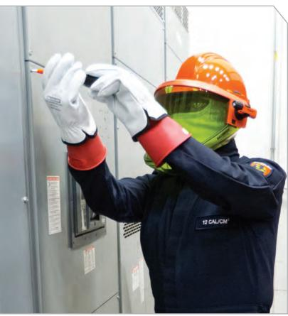
**GLOVE KITS** - Salisbury's insulating rubber gloves are necessary for every electrical worker's complete safety. Salisbury's leather protectors provide needed protection from cuts, abrasions and punctures. To keep these safety items in top condition, proper storage is very important.
